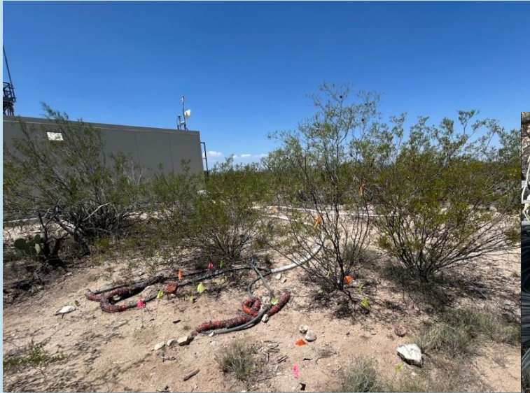
Network of subsurface probes extending from the hut to creosote bushes near the NEON tower
