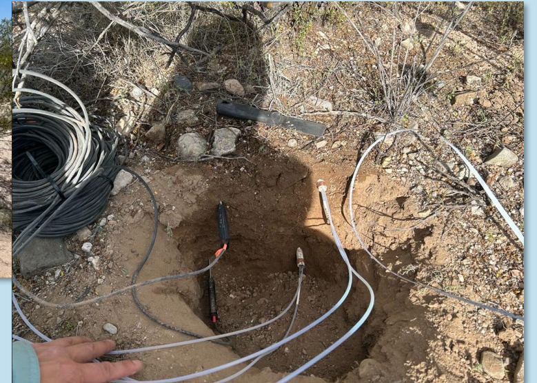
Soil moisture/temp probe (left), VOC probes (right)
